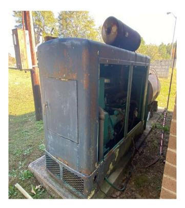
The 1957 generator on the left failed during Hurricane Matthew, leaving the entire Town of Parkton without Wastewater Treatment capacity. Robeson County utilized \$115,000 from NCORR to replace not only the antiquated generator, but also installed automatic transfer switching equipment to restore operations immediately when primary power is lost (see picture on right.)
