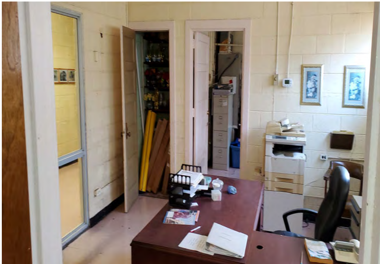
Photograph 8 - Typical Lead-Based Paint on CMU Walls in This One Room Only in Office Area in Main Building.
