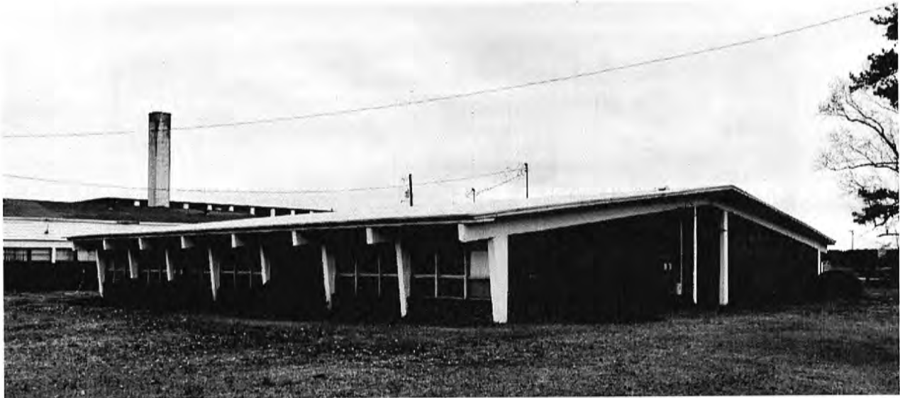
10. 1964 classroom building, northwest oblique (above) and 11. southeast oblique (below)
