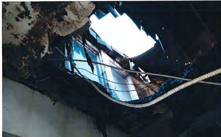
Photo 3: In this interior photograph can be seen an opening in the upper roof, the original clerestory windows, and an opening in the lower (original) roof/ceiling.
