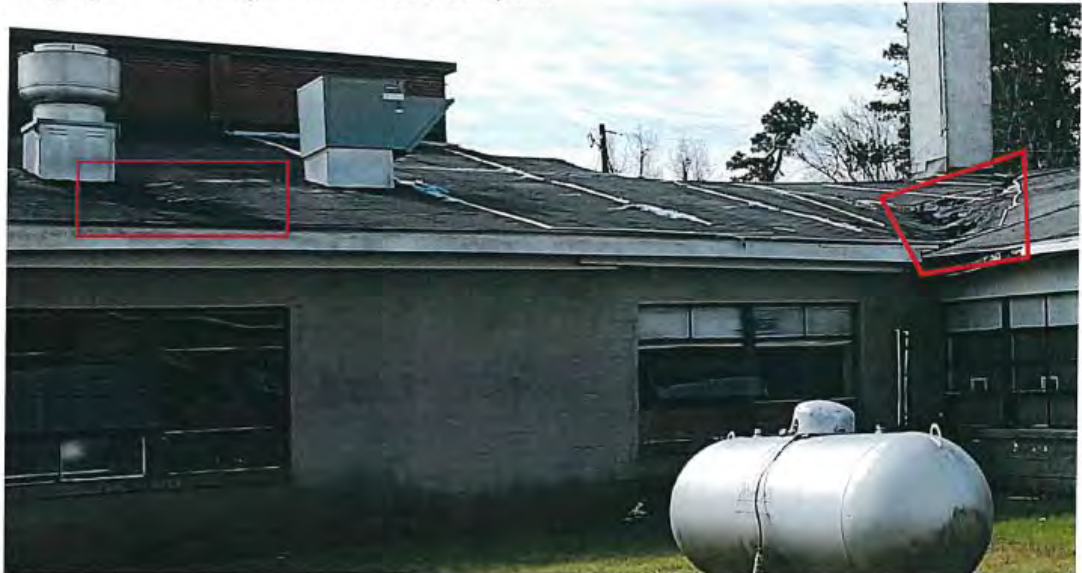
Photo 1: To the right can be seen a collapsed valley. This valley area is highlighted above in the red "diamond" shape. To the left, below the kitchen hood vent, can be seen another opening in the roof. This is highlighted in the diagram above with a red square.
