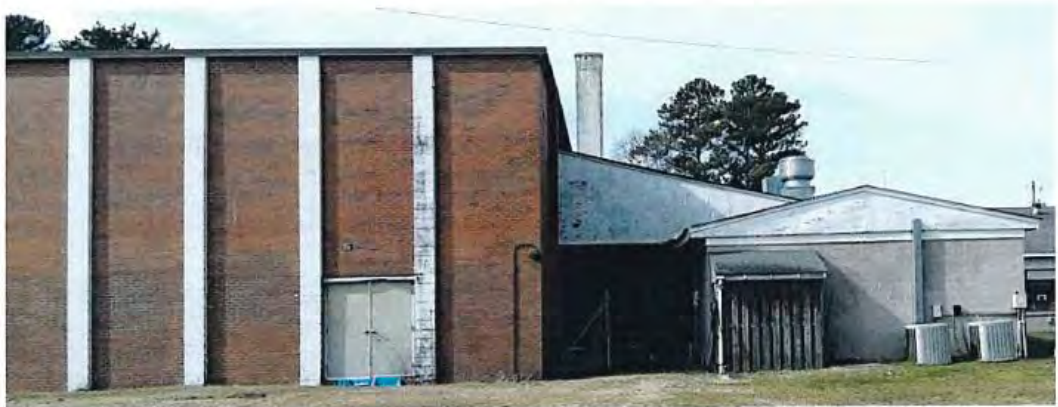
Photo 1: To the right can be seen a collapsed valley. This valley area is highlighted above in the red "diamond" shape. To the left, below the kitchen hood vent, can be seen another opening in the roof. This is highlighted in the diagram above with a red square.
