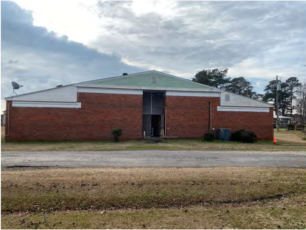
Photograph 7 – Left Side of Classroom Building
