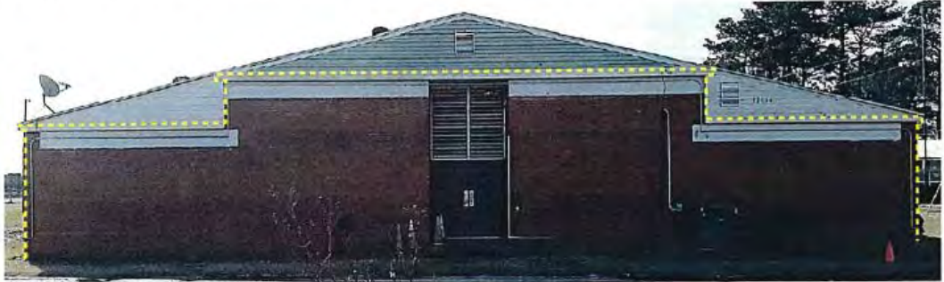
Rear View of the 1963-64 Gymnasium Addition (left) and 2007 Kitchen (right).
