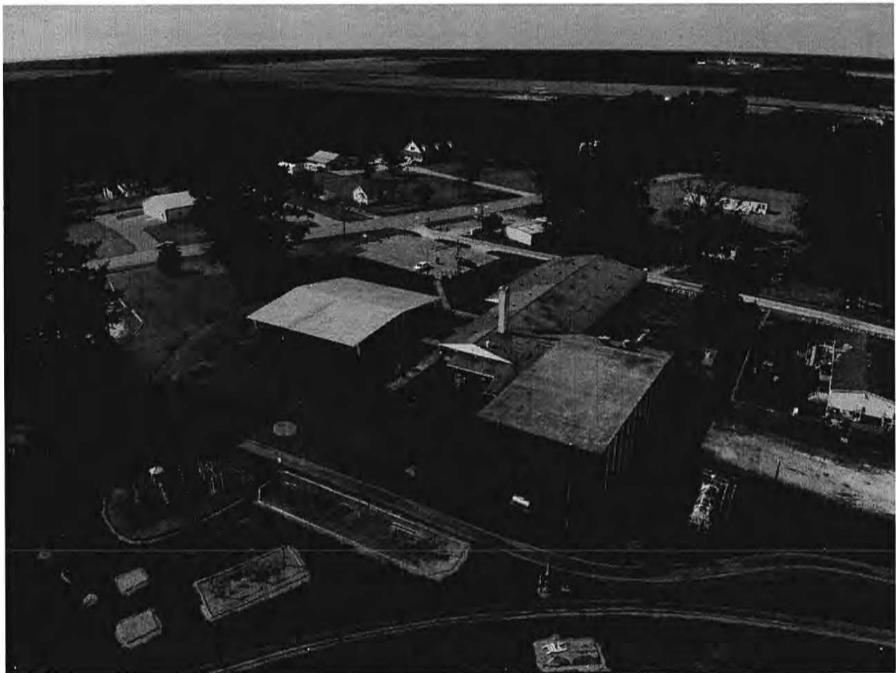
1. Looking northwest from parcel's southeast corner
