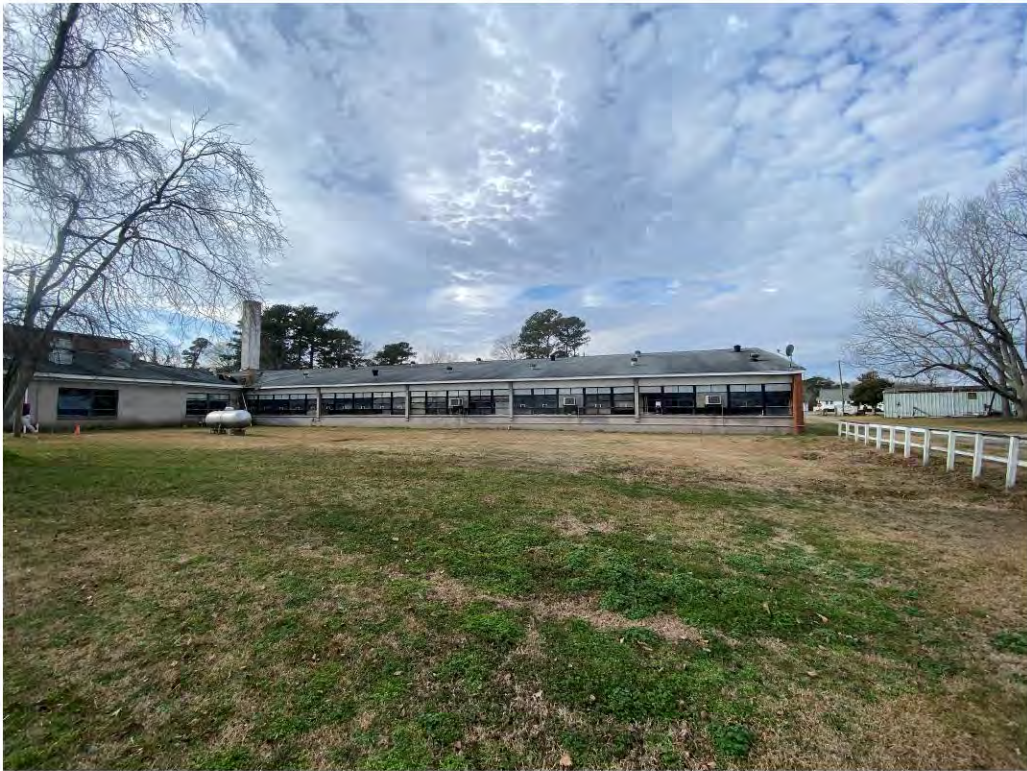
Photograph 6 – Rear Side of Classroom Building
