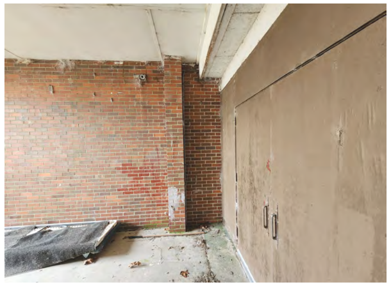
Painted plywood sheathing over masonry veneer.
