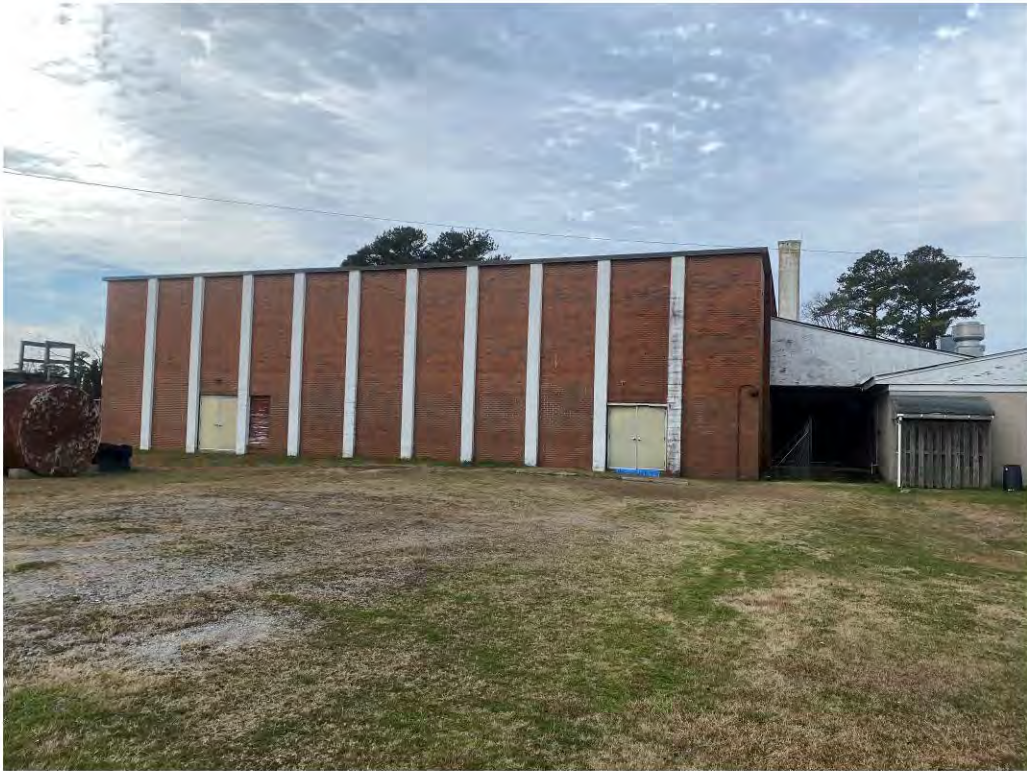
Photograph 4 – Rear Side of Gym
