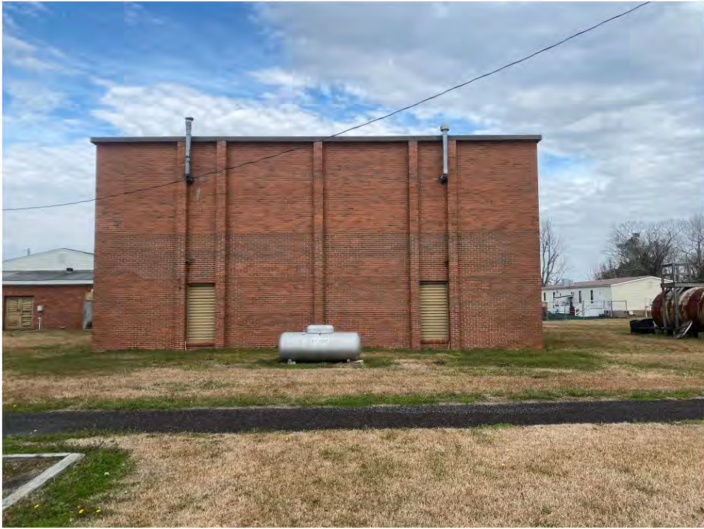
Photograph 3 – Right Side of Gym
