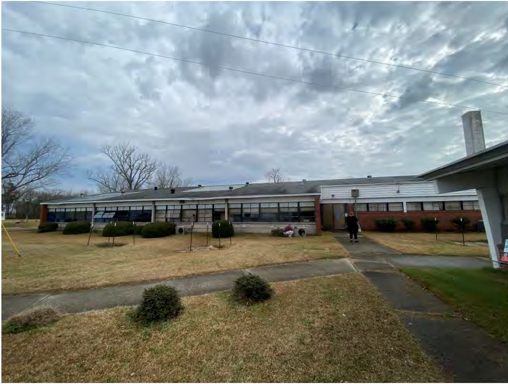
Photograph 1 – Front View – Classroom Building
