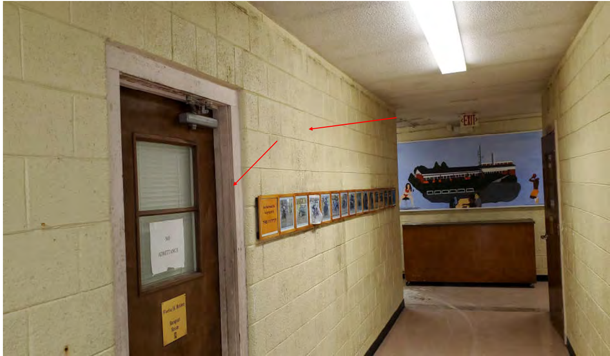
Photograph 9 - Typical Mold Growth on Walls, Door Components, & Other Surfaces Located Throughout the Main Building.
