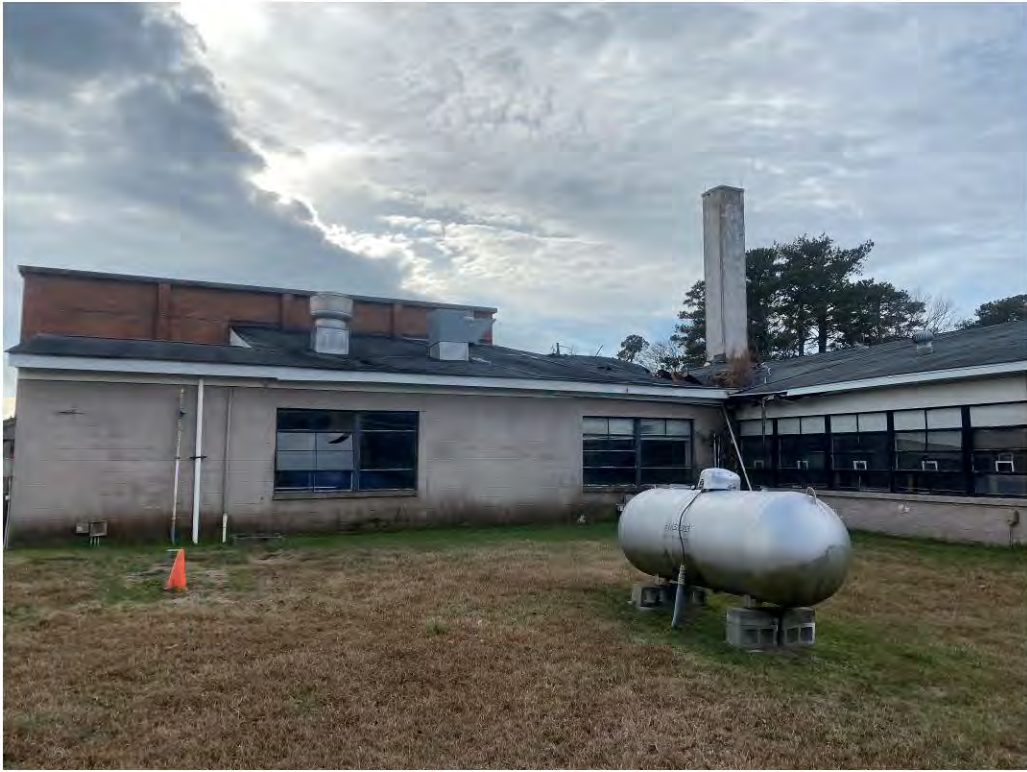
Photograph 5 – Left Side of Gym/Connector
