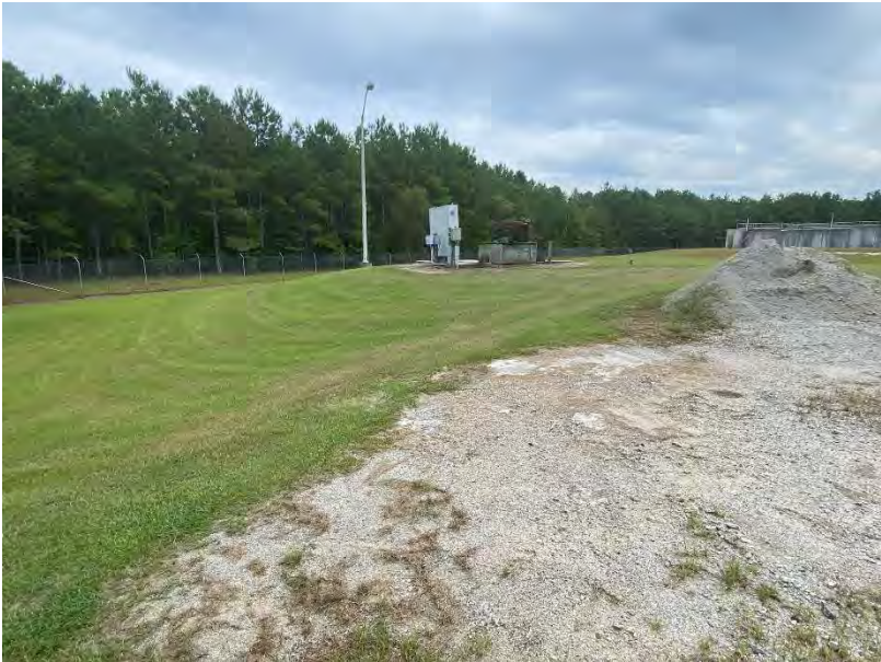
Photo No. 10 Lift Station
