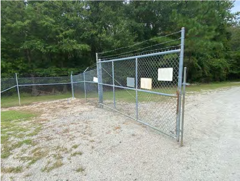
Photo No. 8 Entry Gate System
