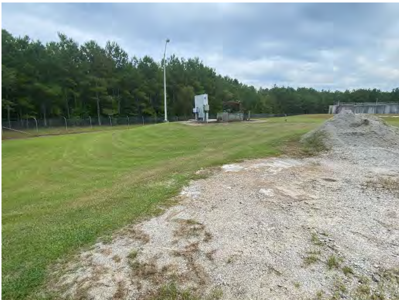
Photo No. 10 Lift Station
