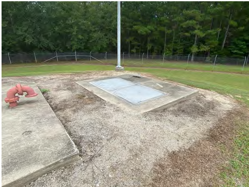
Photo No. 14 Lift Station Equipment Access
