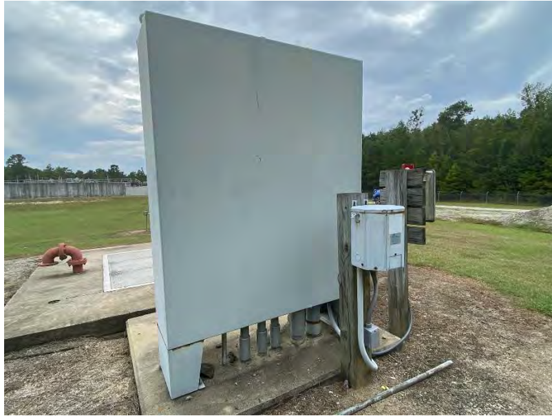
Photo No. 13 Lift Station, Facing WWTP
