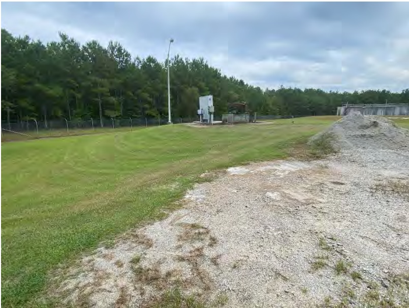
Photo No. 10 Lift Station
