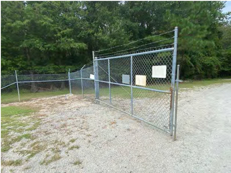
Photo No. 8 Entry Gate System
