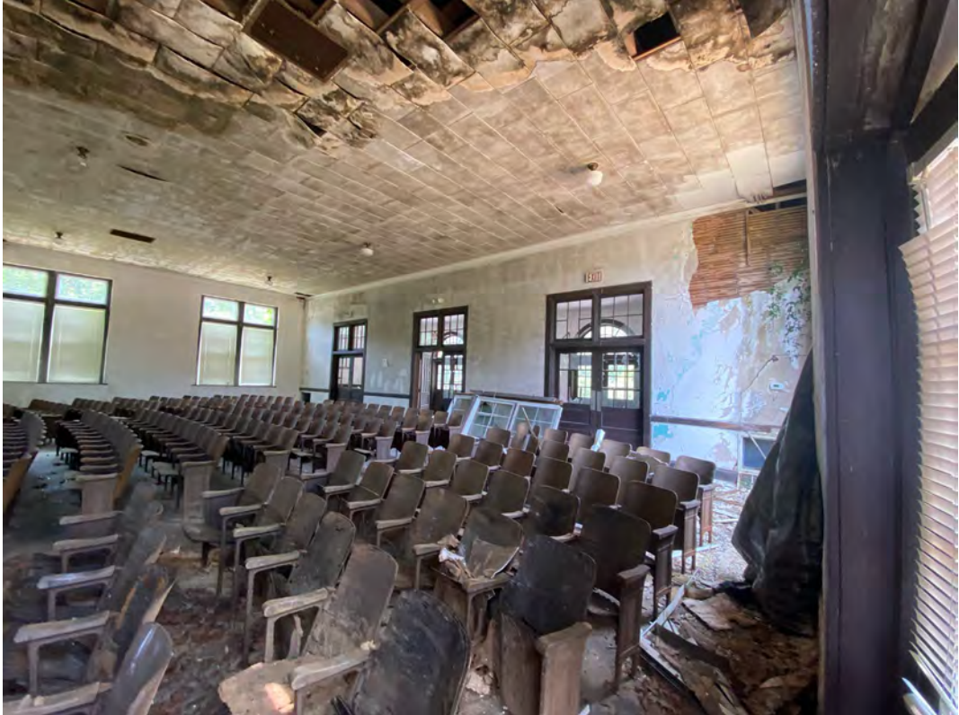
Site Visit Photos May 26, 2021 - Town of Magnolia Auditorium, Duplin County, NC
