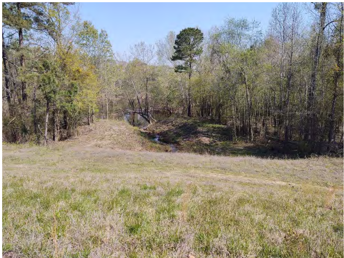
RS – 251201 – Top of Levee Looking North Toward Tar River
