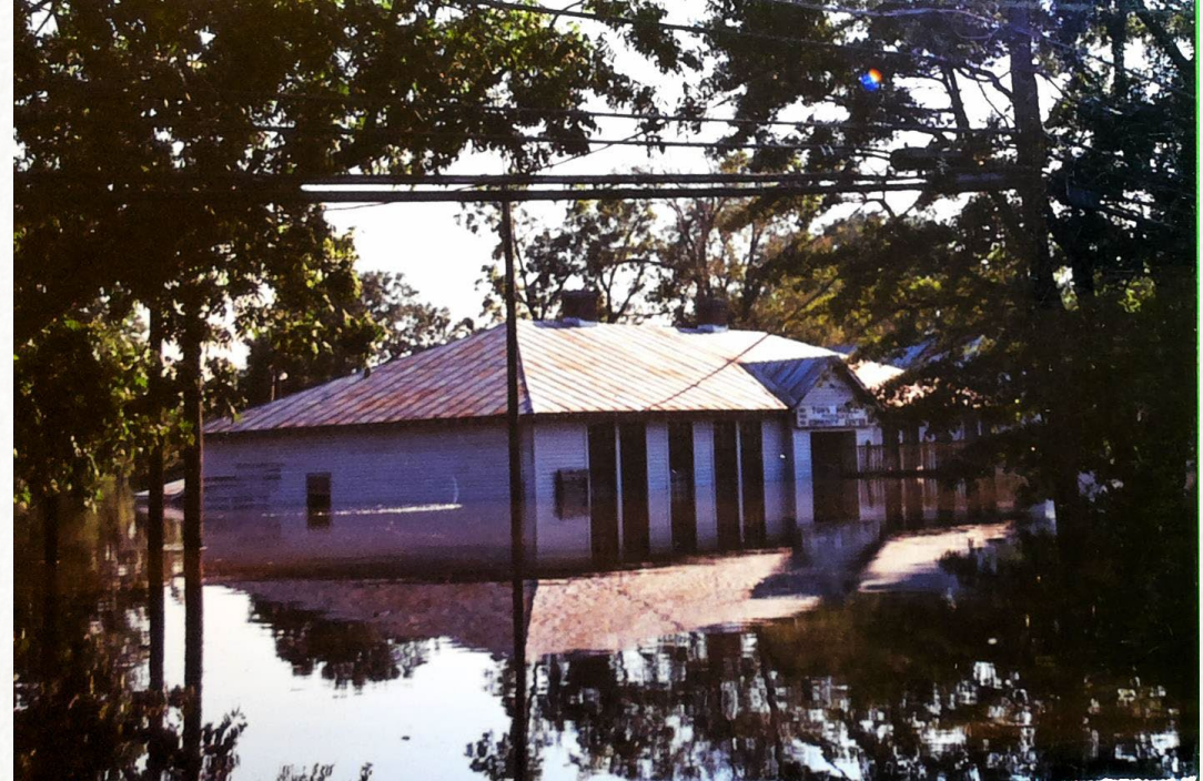
Princeville Town Hall (1999) following Hurricane Floyd.
