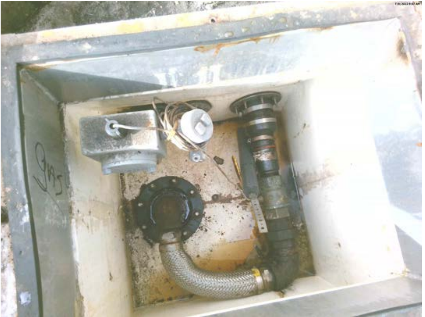
PICDIAG REGULAR TANK TOP SUMP
