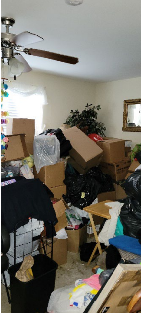
Excessive contents in various locations throughout the unit obstructing the visual inspection
