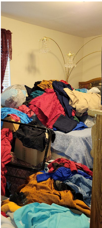
Excessive contents in various locations throughout the unit obstructing the visual inspection
