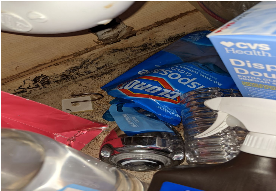
Apparent water damage and suspect visible mold growth within the bathroom cabinet
