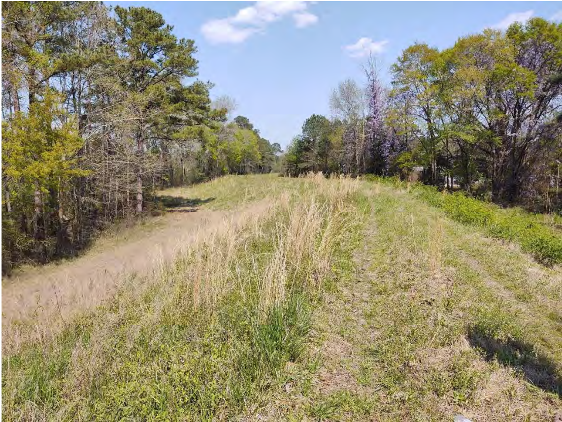
RS 250294 – Top of Levee Looking East
