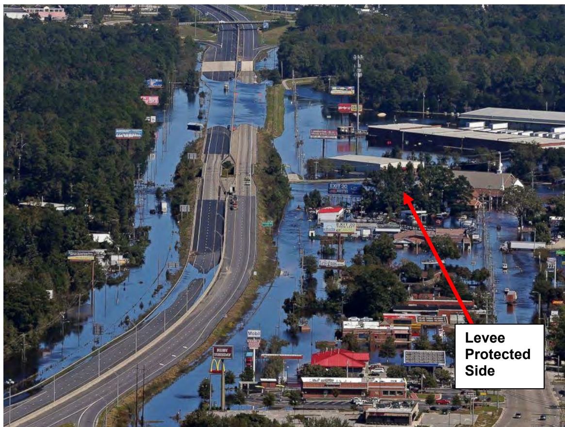
Figure 2-2. Flooding along I-95 and inside the Lumberton Levee from Hurricane Matthew; area to right of road is the levee protected side of Lumberton (Source: City of Lumberton).
