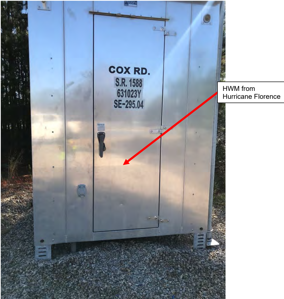
Figure 3-9. Example of HWM from Lumberton field visit near the VFW Road and railroad intersection by the flood gate location.
